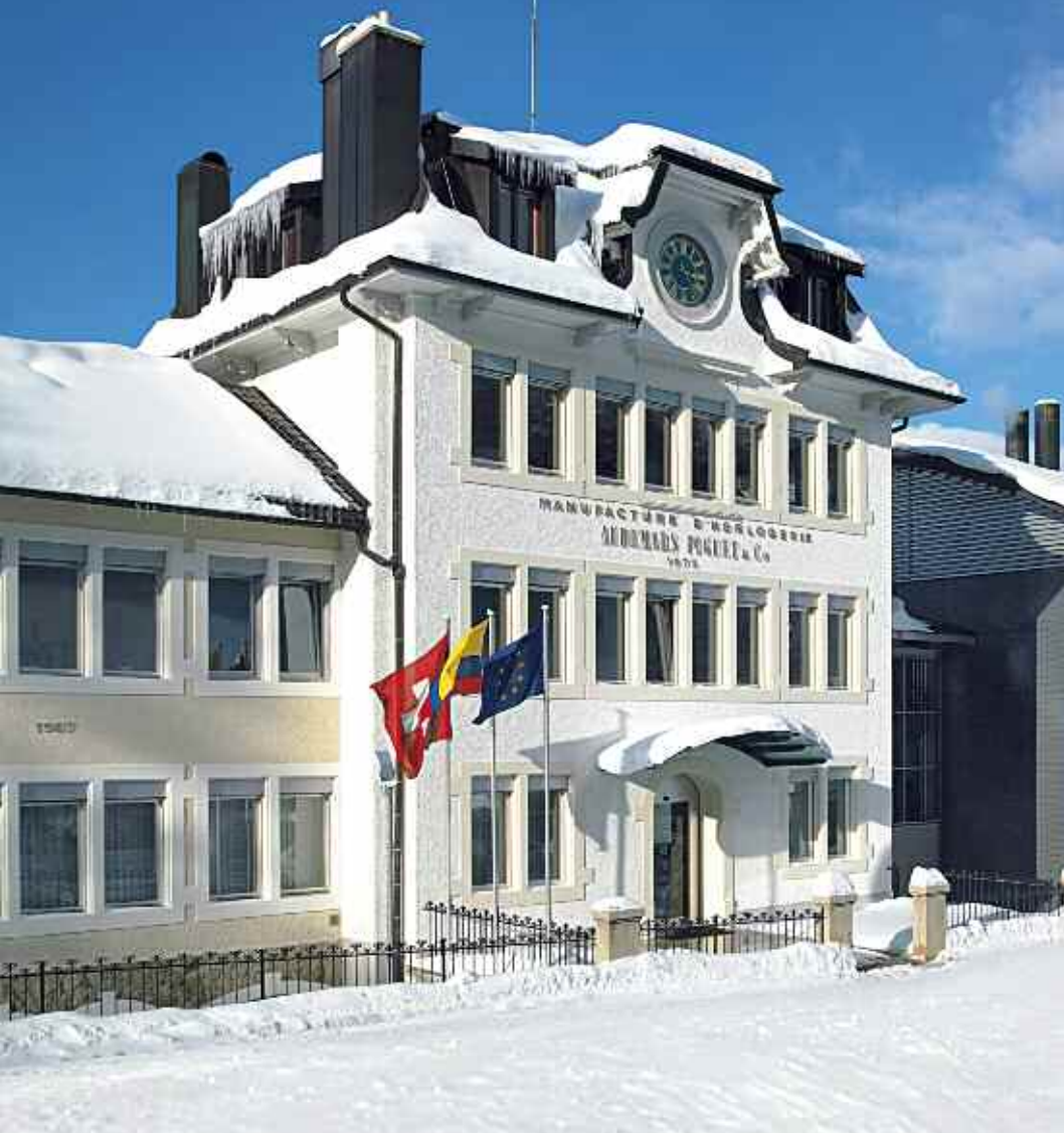
AP's headquarters and factory on Route de France
